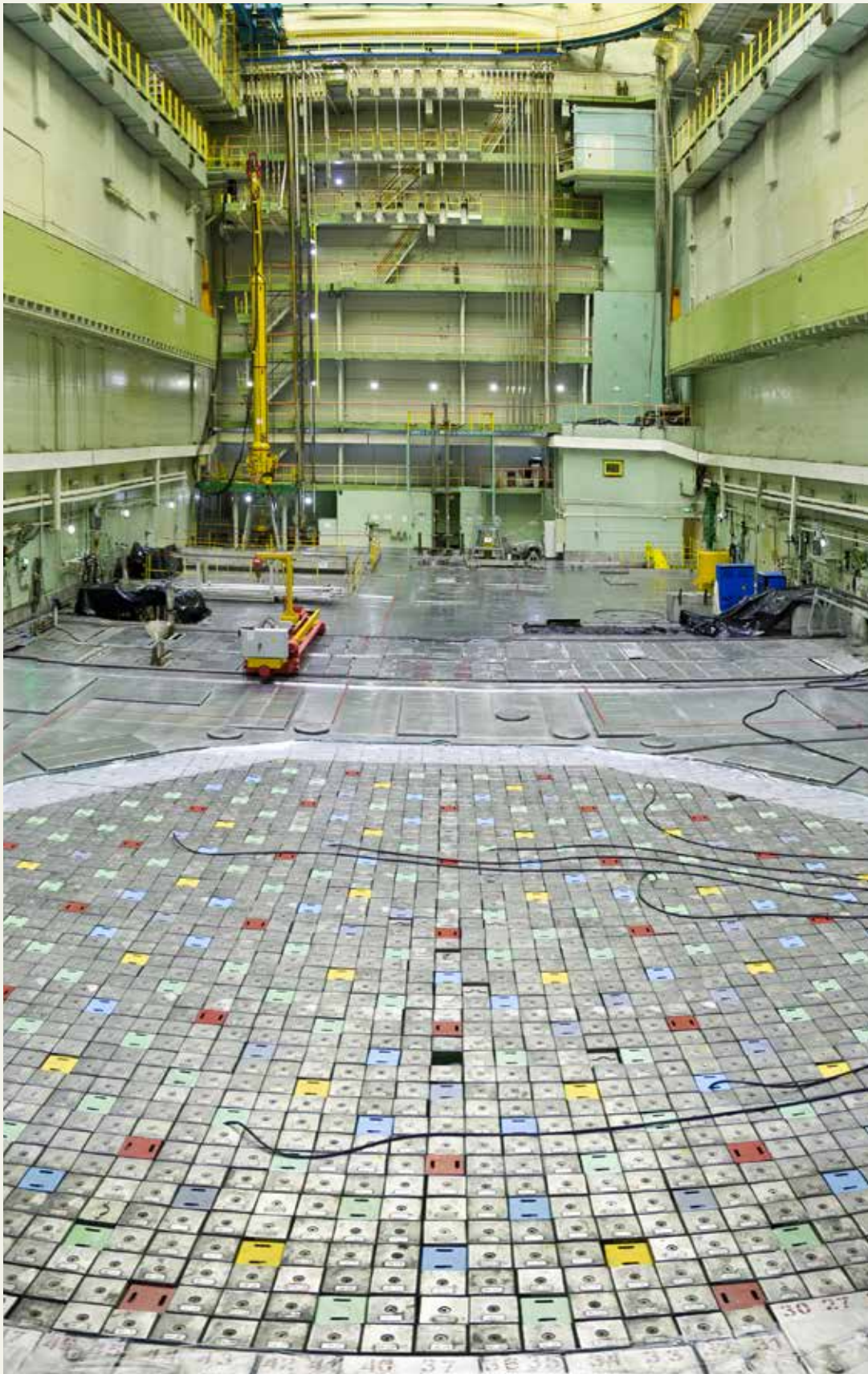
The central hall of a Russian nuclear reactor showing the reactor lid during maintenance and replacement of the reactor fuel elements.
